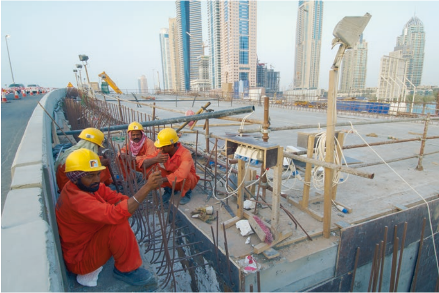
Fig. 3.7 Construction workers in Dubai, United Arab Emirates (Credit: tanukiphoto © istockphoto)
