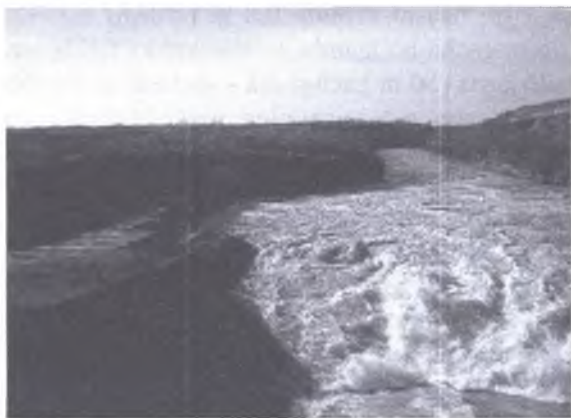
13.18 - rasm. Qiyshiq gidravlik sakrash oqibatida inshoot pastki hefini yuvilishi.
