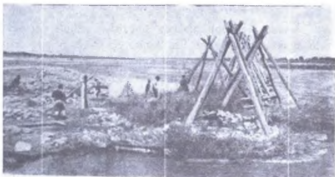
1.8 - rasm. Daryo o'zaniga sepoya o'rnatish.
