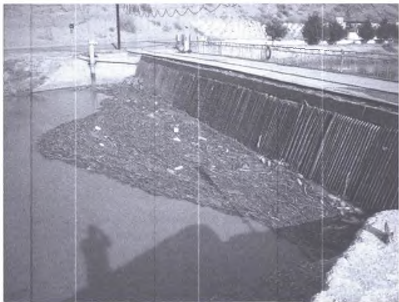
8.8 - rasm. Qo'qim ushlovchi panjaralar
